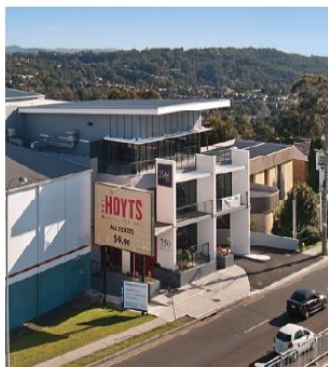
FRONT VIEW OF JSA GROUP
